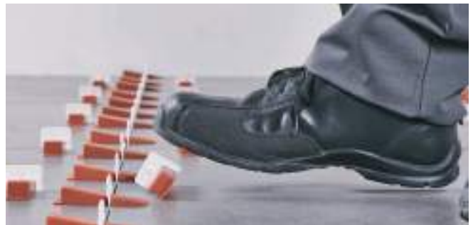
REMOVE CLIP AND WEDGE
