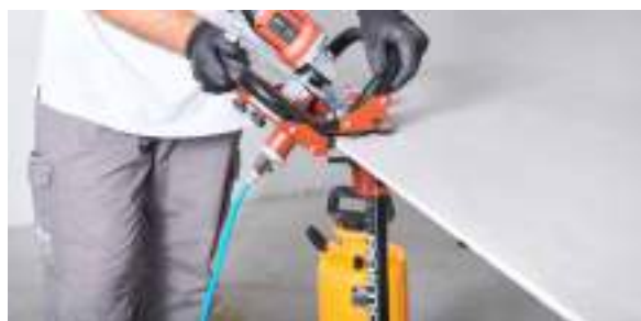
WATER COOLING TANK
